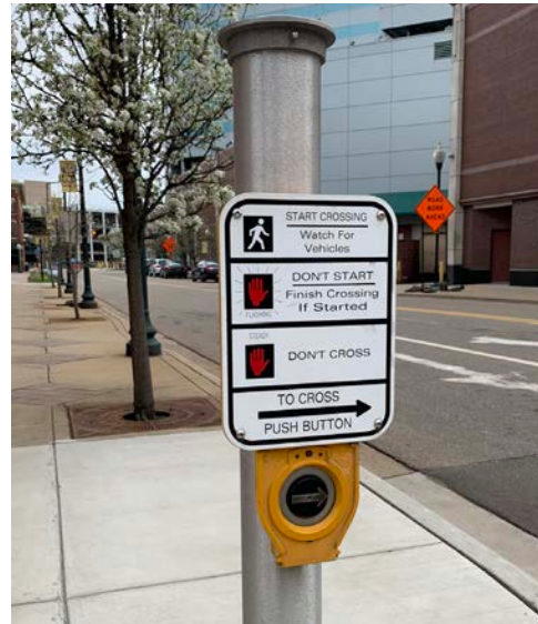
Example of an accessible push button for an actuated crosswalk
