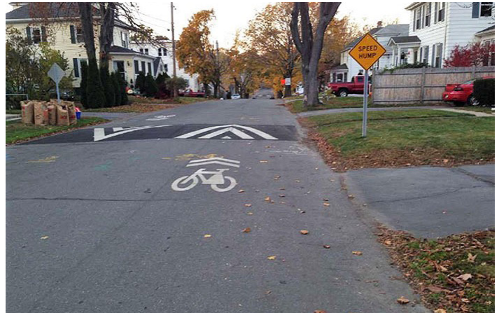
Speed Hump (in asphalt) Source: FHWA / Lucy Gibson
