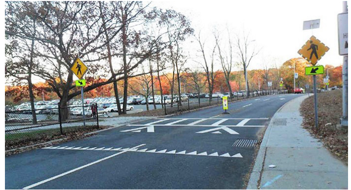
Speed Table (in asphalt) with Mid-block crossing
