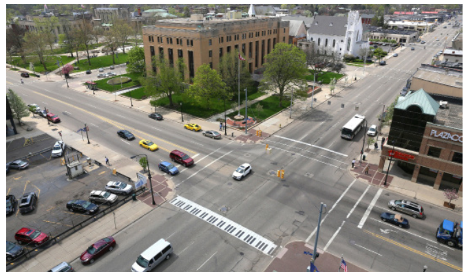
Downtown Intersection. Photo credit: MLive
