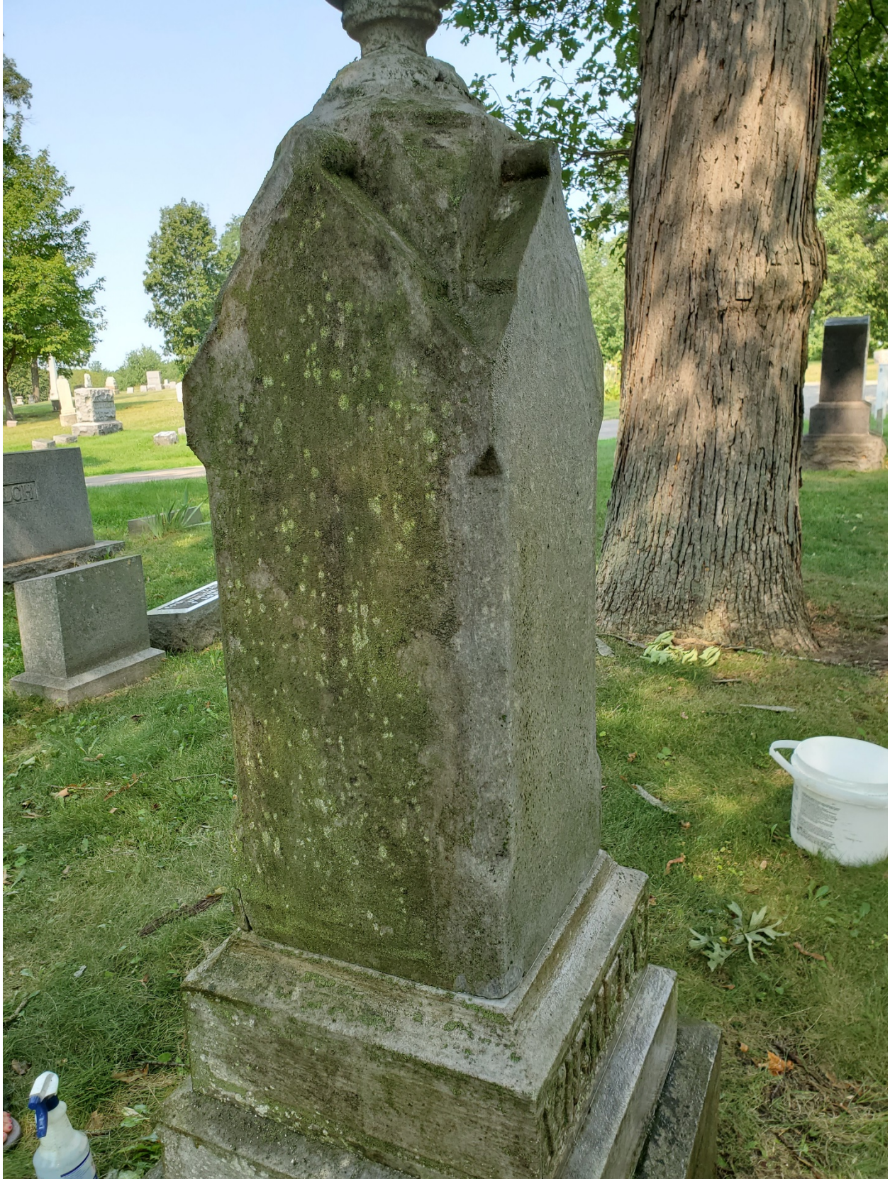
The obelisk is untouched on the left and scrubbed on the right.
