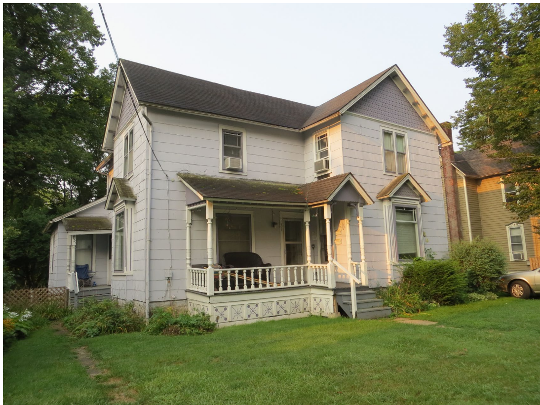
731 Minor Transite (cement- asbestos) siding Original porch skirt and posts
