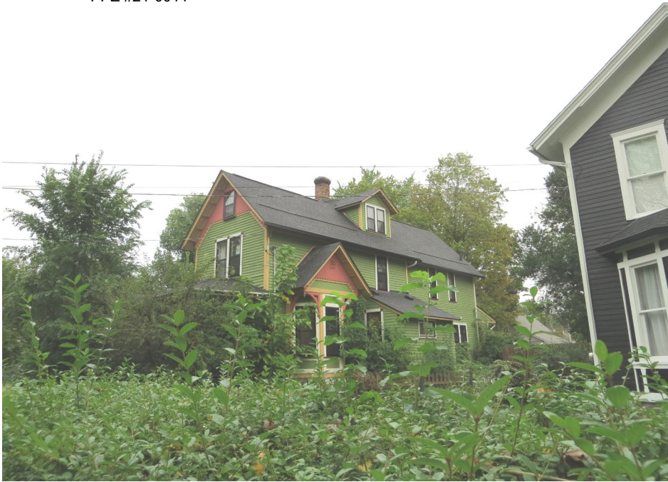
(1) 911 S. Park – Oct. 12, 2021 – southwest corner from the sidewalk (3) South side looking northeast
