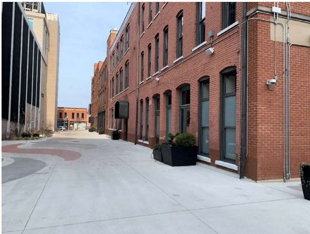
1.) 251 E Michigan – Northwest Corner
