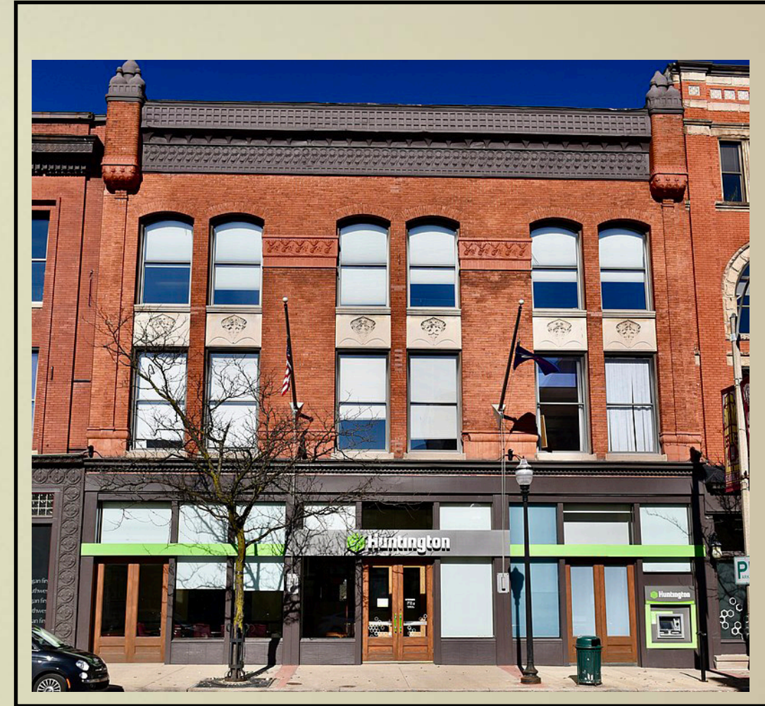
Desenberg Building - South facade current condition Photo Credit: Jim Roberts Source: Wikipedia.com
