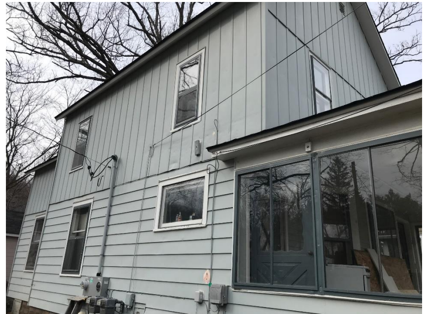
4.) 908 Village – South East Corner – fixed pane window
