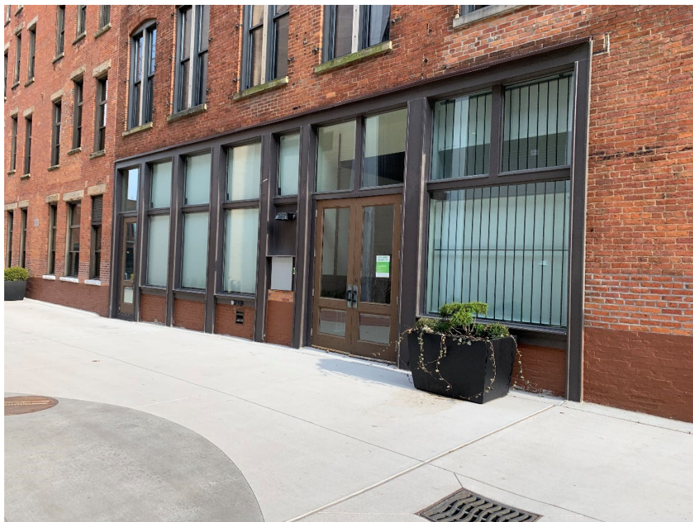
3.) 251 E Michigan – Existing Storefront on North Face
