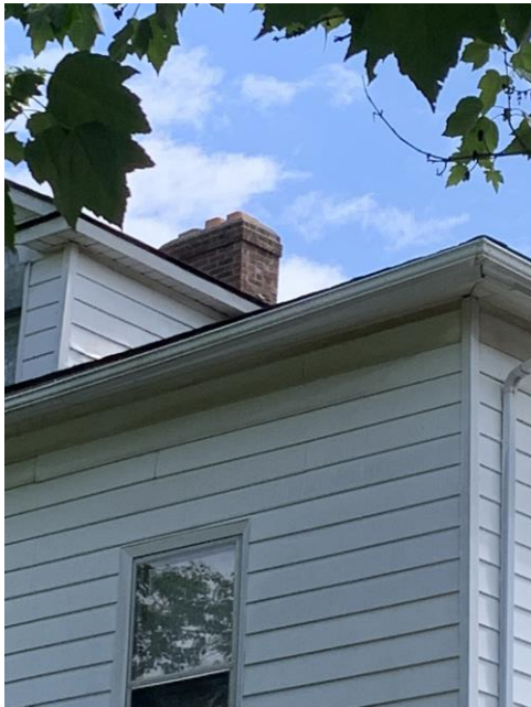
(3) Southwest corner, looking northeast, chimney detail
