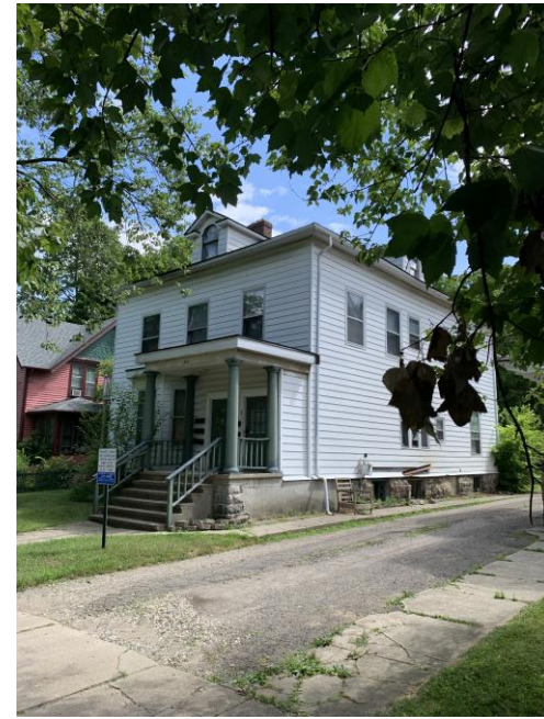
(2) Southwest corner, looking northeast
