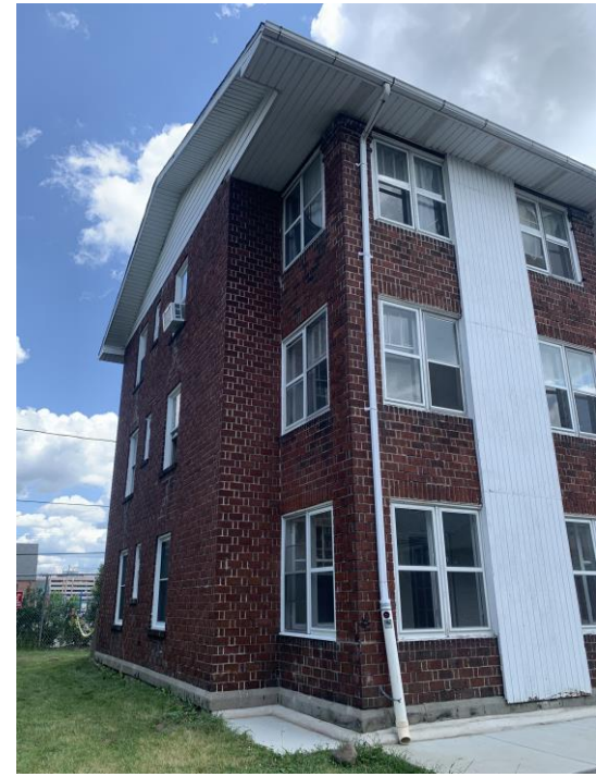
(2) Northwest corner, looking southeast
