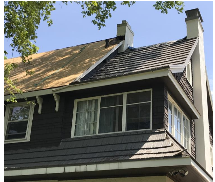
(4) Rear, looking northeast. Chimney detail
