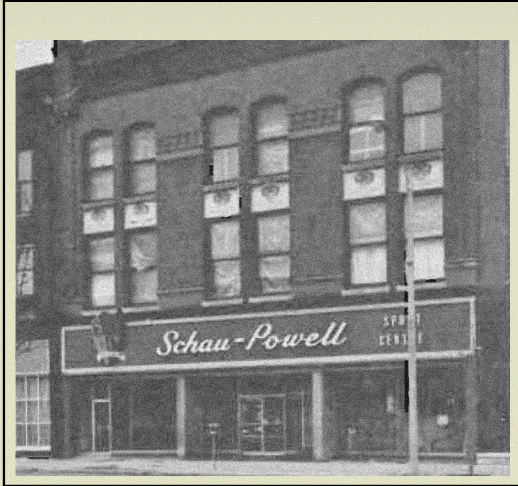
Desenberg Building - South facade 1979. Photo Credit: Unknown Source: Walking Through Time
