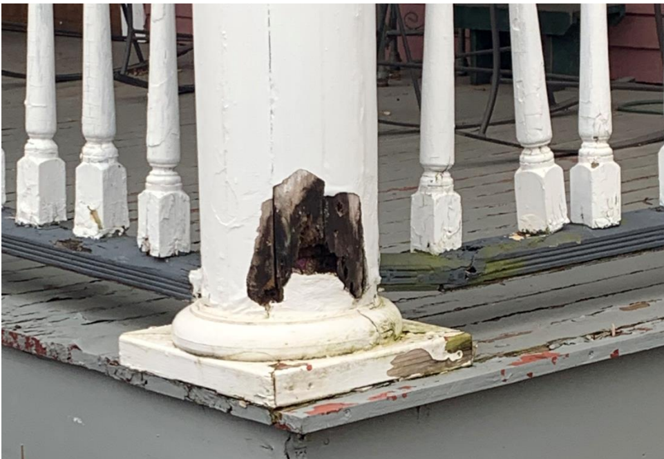
(1) 511 Woodward – East Face of building (3) North column deterioration detail
