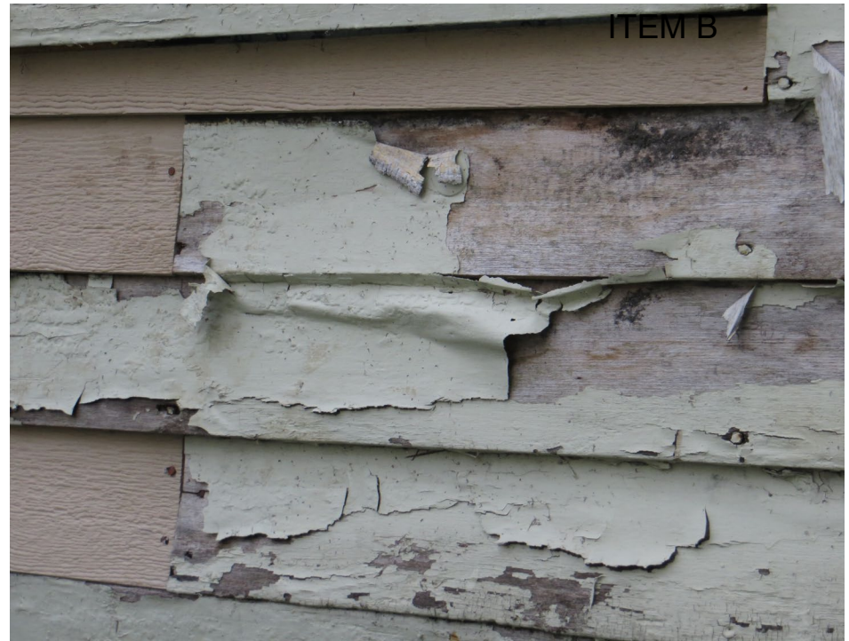
(2) W side typical peeling paint & replacement siding (4) North front, 2 nd & 3 rd floor peeling paint
