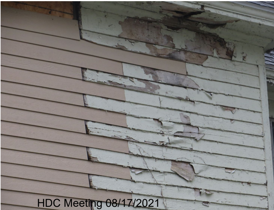
(1) 207 W. Vine – August 12, 2021 – E side (3) West side peeling paint, soffit & replaced siding
