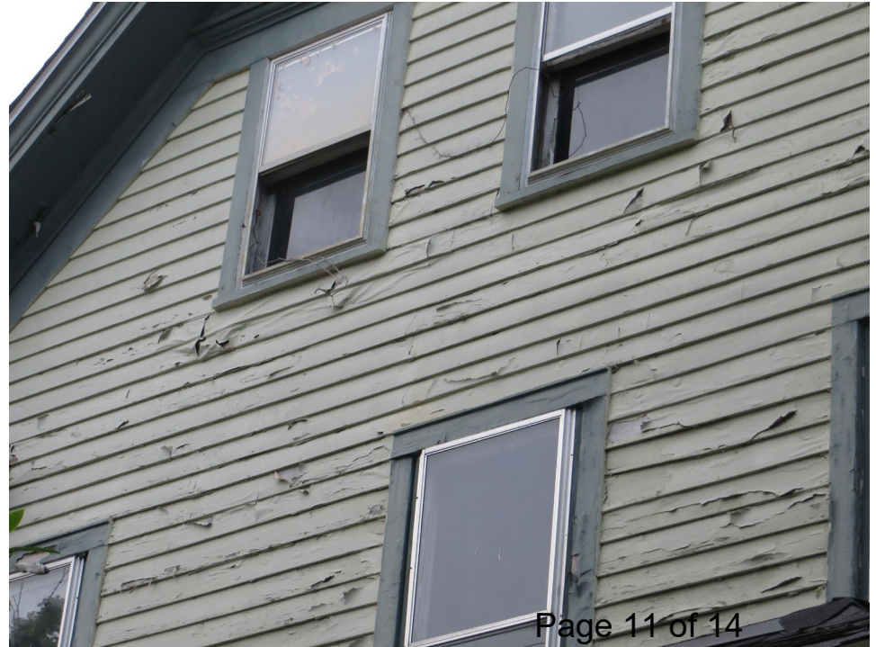
(2) W side typical peeling paint & replacement siding (4) North front, 2 nd & 3 rd floor peeling paint
