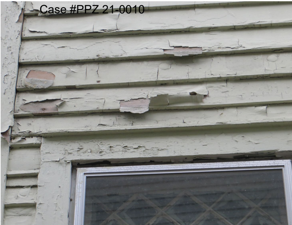
(1) 207 W. Vine – August 12, 2021 – E side (3) West side peeling paint, soffit & replaced siding
