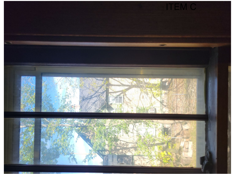
(2) Typical windows – upper sash with ribbon lites
