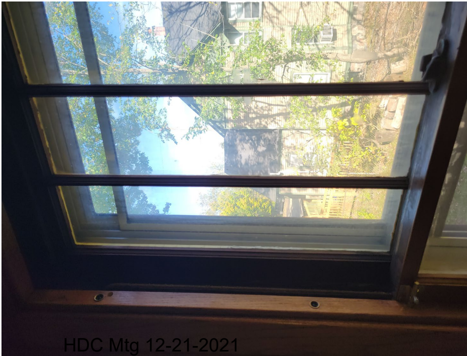
(3) Typical windows – upper sash with ribbon lites
